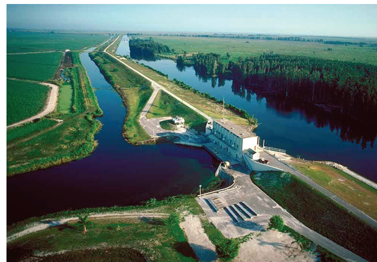
Figure 1.11. Pump station on a drainage canal in southern Florida (South Florida Water Management District).
