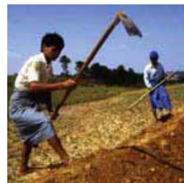
Farmers working on the construction of contour bunds, Myanmar
