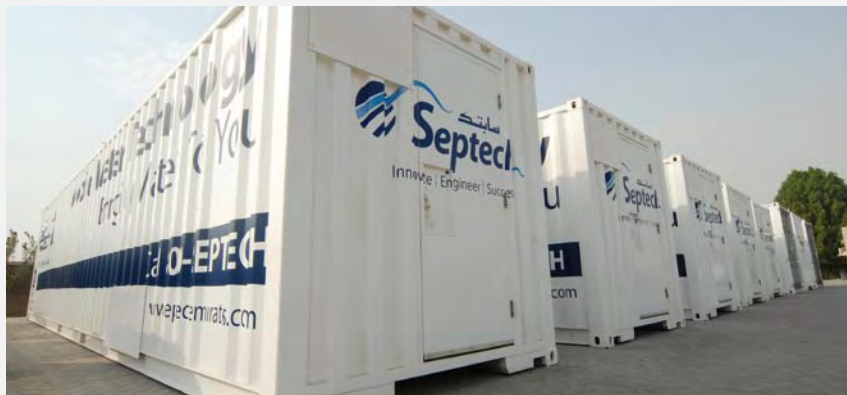
The 12-metre mobile containers can produce 1,000m 3 of water each day
